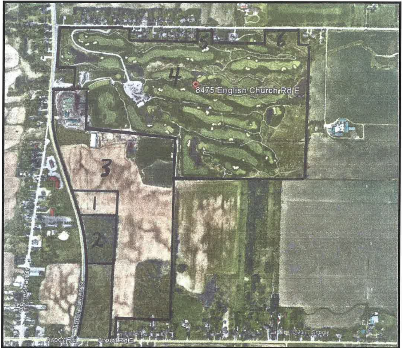
FIGURE 1.b: AERIAL PHOTOGRAPH OF THE SUBJECT AREAS SHOWING THE LAND PARCELS (LOTS 1 TO 5) DISCUSSED IN THIS REPORT
