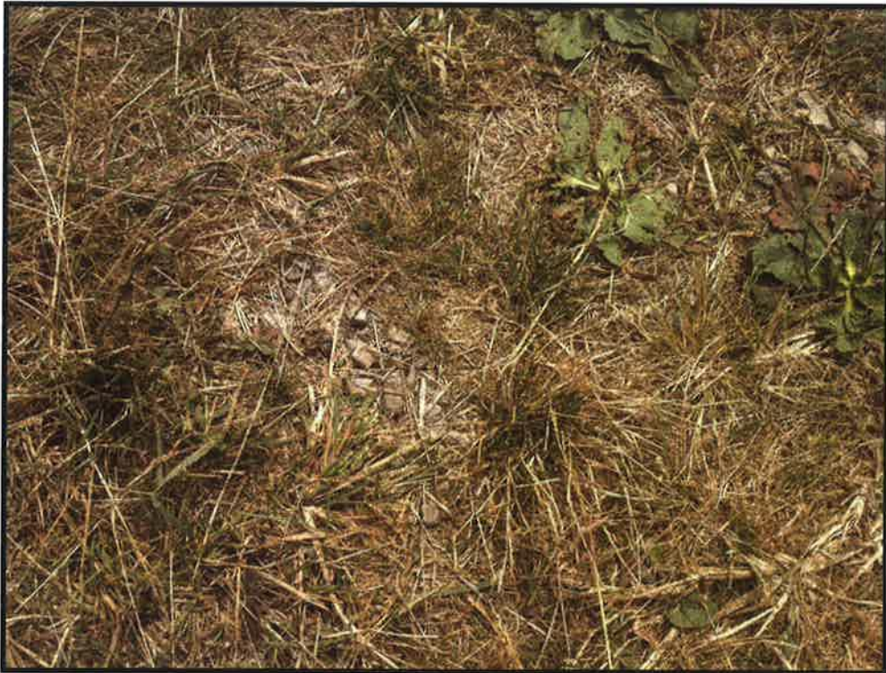
Image 8: East Parcel (Part 6) Gravel and Subsoil Visible on Surface Facing North
